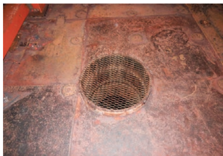
Typical hot gas recirculation pipe
