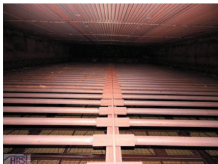
Typical ammonia injection grid
