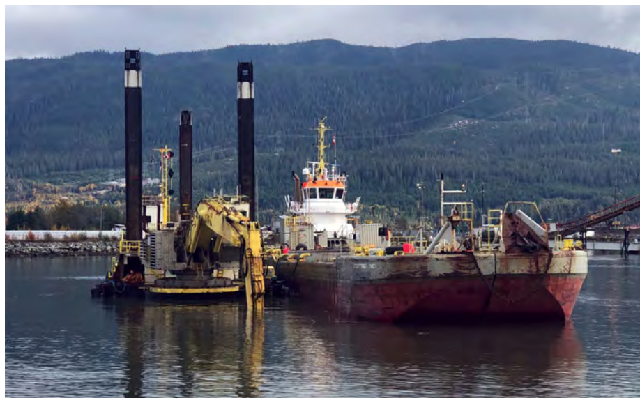
Dredging at the marine offloading facility in the Douglas Channel in British Columbia as part of repurposing the wharf so it can receive LNG carriers
