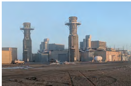
Sask Power Ermine plant uses two clutched LM6000s to provide both real and reactive power to the Saskatchewan grid.
