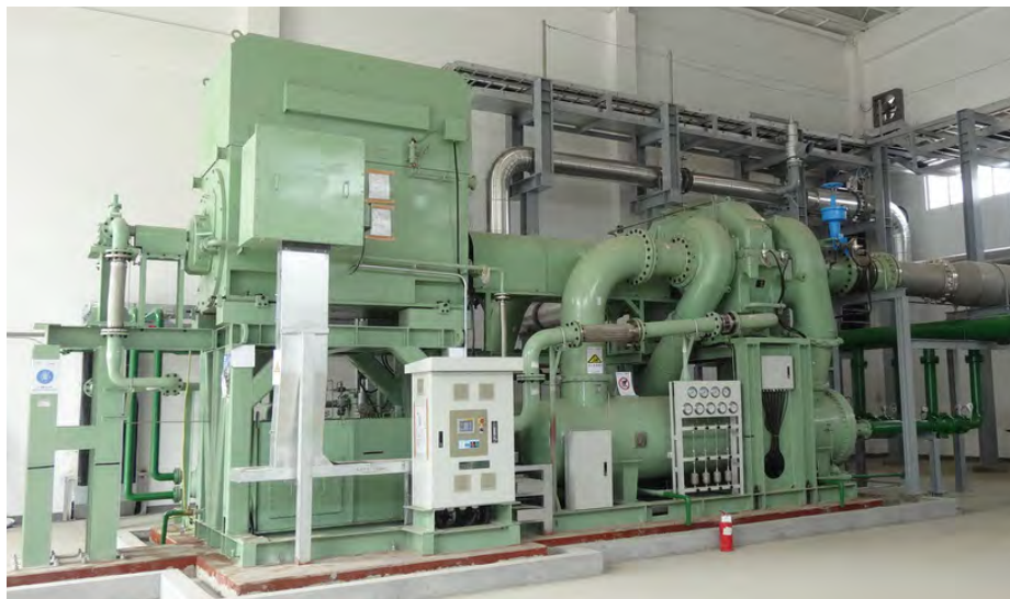
Sullair centrifugal installation
