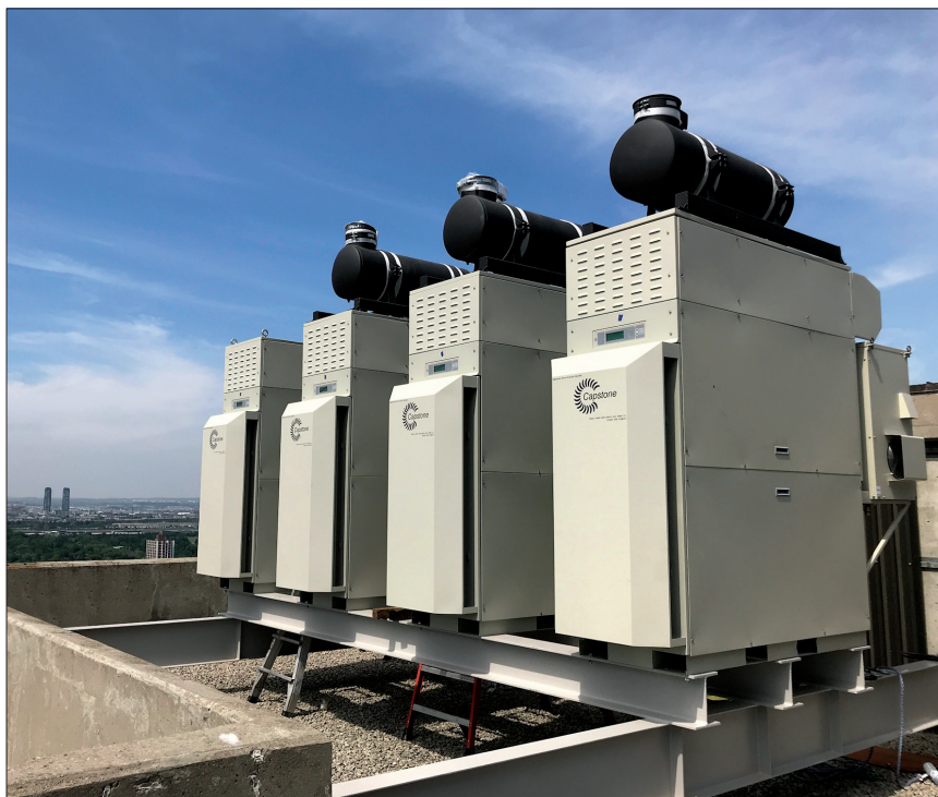
A group of Capstone C65 microturbines on a rooftop in Canada, powering an apartment building.
